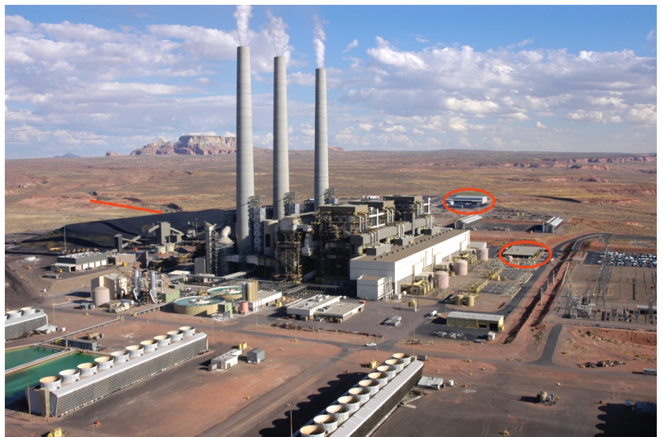
The NGS site as it was in November 2019 when operations ceased. The only visible assets remaining are the Administration Building and Warehouse in red circles, and railroad, red line at left.
